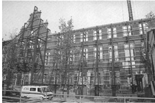
Figure 2.9 Façade conservation, Amsterdam
